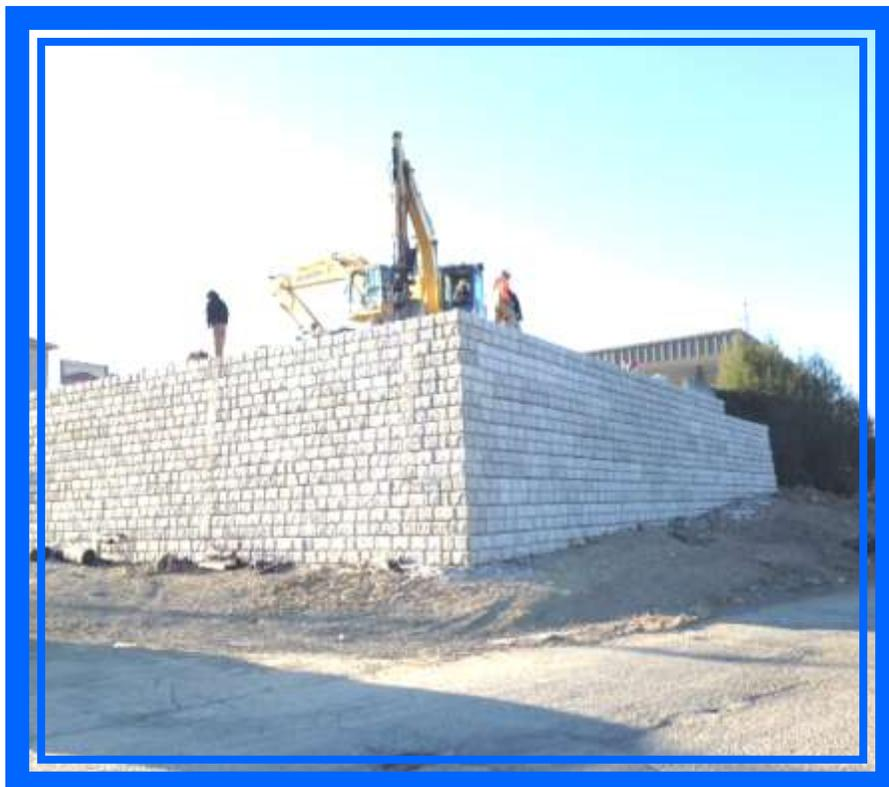
Contractors were on site at the beginning of November to start demo of the existing wall at the Merchant Street facility. Upon completion of the demo work began by setting redi-rock. The project was completed in mid January.
