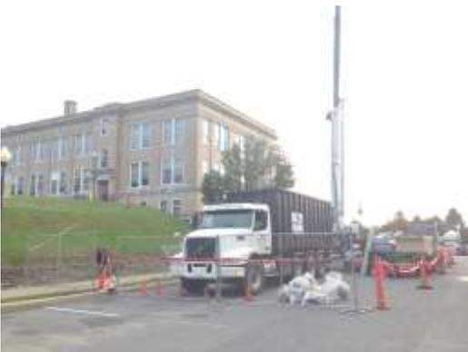
September 26th Mansuetto & Sons began work on the Jaynes Hall roof. The old roof materials were demoed and removed quickly so that the new material could be placed. The contractor also insulated exterior duct work on air handler units. The new roof is an Ethylene-Propylene-Diene-Monomer (EPDM) rubber. The roof was completed in mid November.
